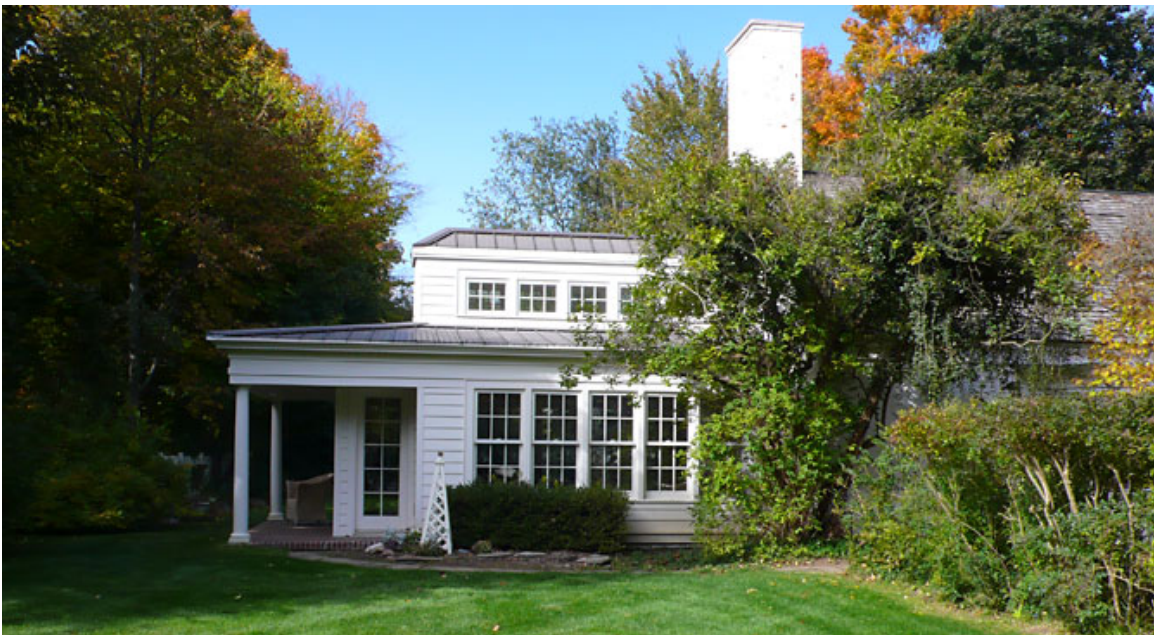
Side View of New Sunroom Exterior
